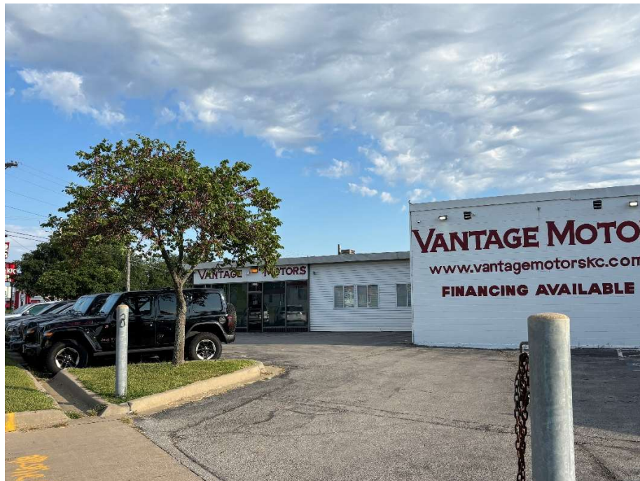
Figure 2. Front of Building 8-28-26
