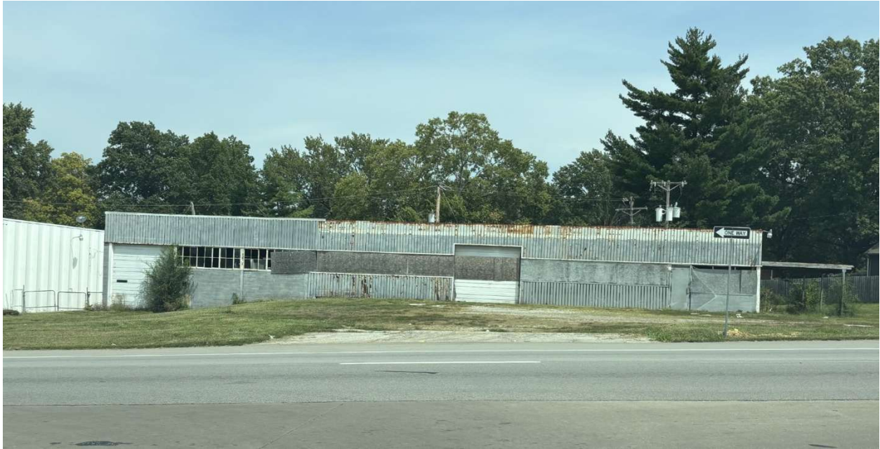
Figure 9. Building located on adjacent parcel, 10016 E 350 Hwy, owned by same property owner.
