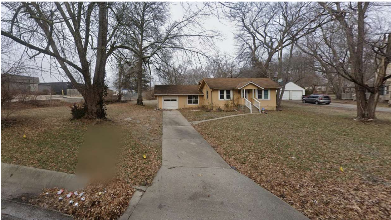
Facing 6920 Laurel Ave. (vacant residence)
