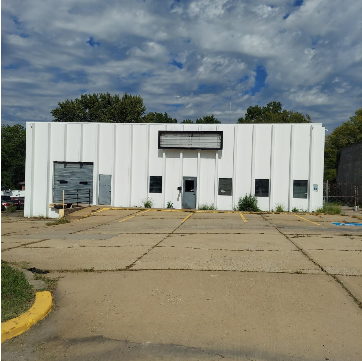
The building located at 10012 E 350 Hwy
