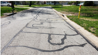
Street Crack Sealing
