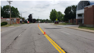
Pavement Marking Project
